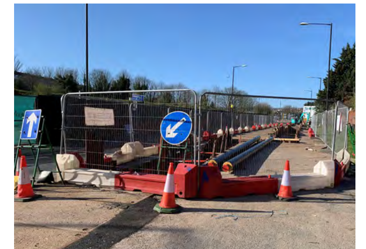
Installation of Bedminster heat network
