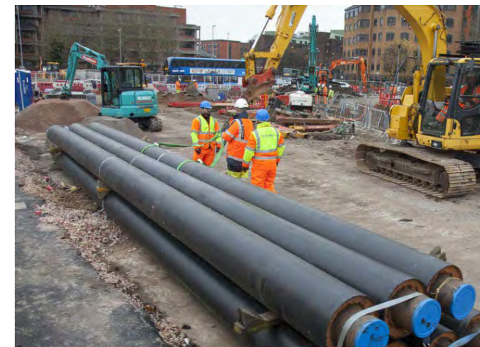
Installation of Redcliffe heat network
